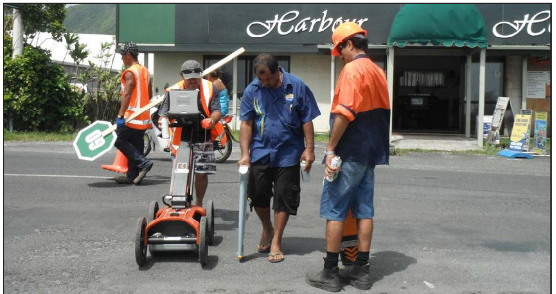
Contractors using the portable ground penetrating radar on the main road in Avatiu
